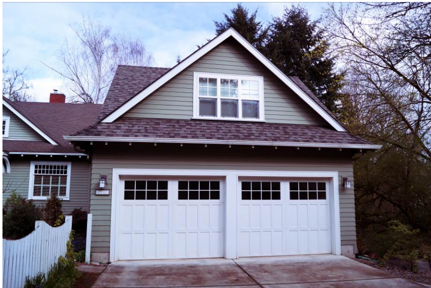
Figure 6. Looking north at the south façade of garage. August 2014.
